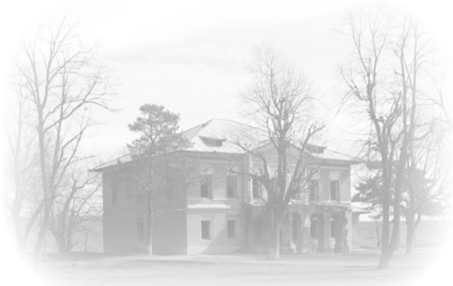
The picture shows the family's domain at Soleshtiu its current state of deterioration today, where both letters from this lot have been addressed to.
